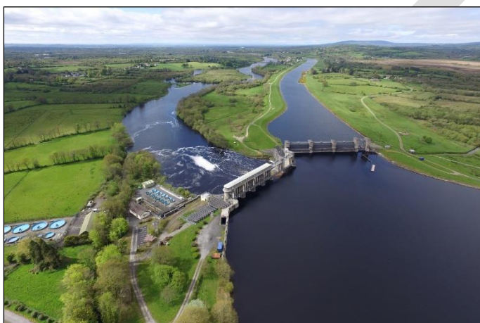
Plate 2 Parteen Regulating Weir with the old River Shannon (left channel) and headrace canal visible.
