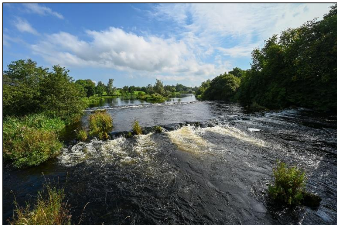
Plate 10 Looking upstream from the Castleconnell footbridge, August 2021 (Site 1).
