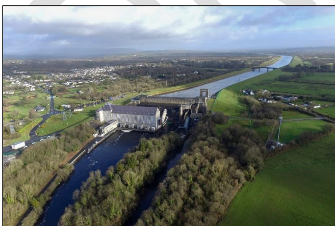
Plate 3 Ardnacrusha hydroelectric station with the headrace canal also visible.
