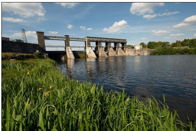
Plate 1 Parteen Regulating Weir located upstream of the study area. Up to 97% of the water in the Lower River Shannon SAC is abstracted at this point to fuel Ardnacrusha hydroelectric station.
