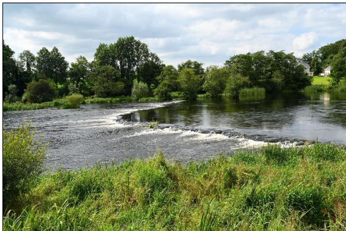
Plate 49 Lower River Shannon at Site 6 showing one of the artificial fisheries weirs installed by the ESB. This one is known as “Pa’s Gap”.
