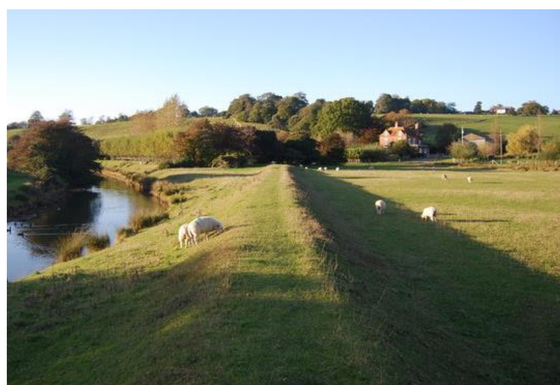
Example of flood embankment (River Tillingham) (Image copyright: N Chadwick under the licence Creative Commons – Attribution-ShareAlike 2.0 Generic – CC BY-SA 2.0)
